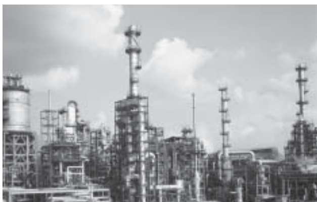
PX-PTA plant of Panipat Refinery.
