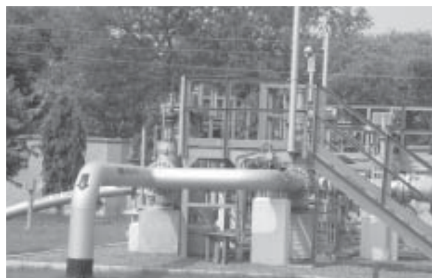
An installation of Panipat-Bhatinda pipeline.
