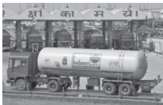
An Indane bottling plant
