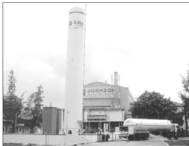
"LNG at the Doorstep" through cryogenic tankers for consumers located away from gas pipelines.
