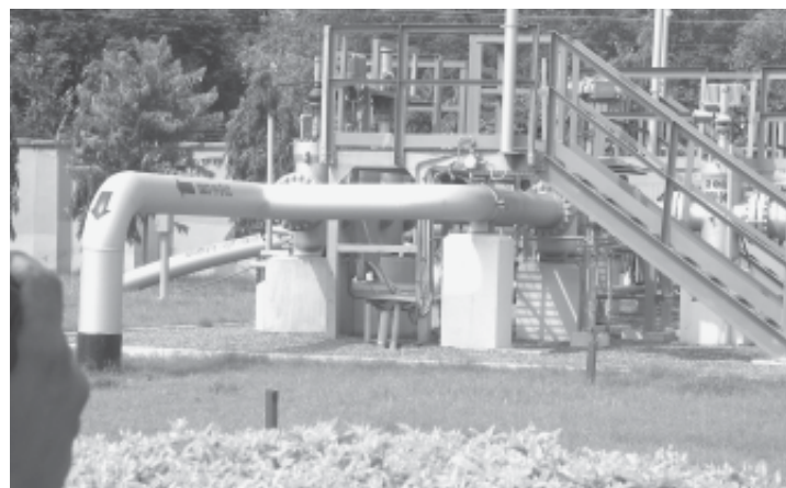
Transporting cost effectively to consuming centres
