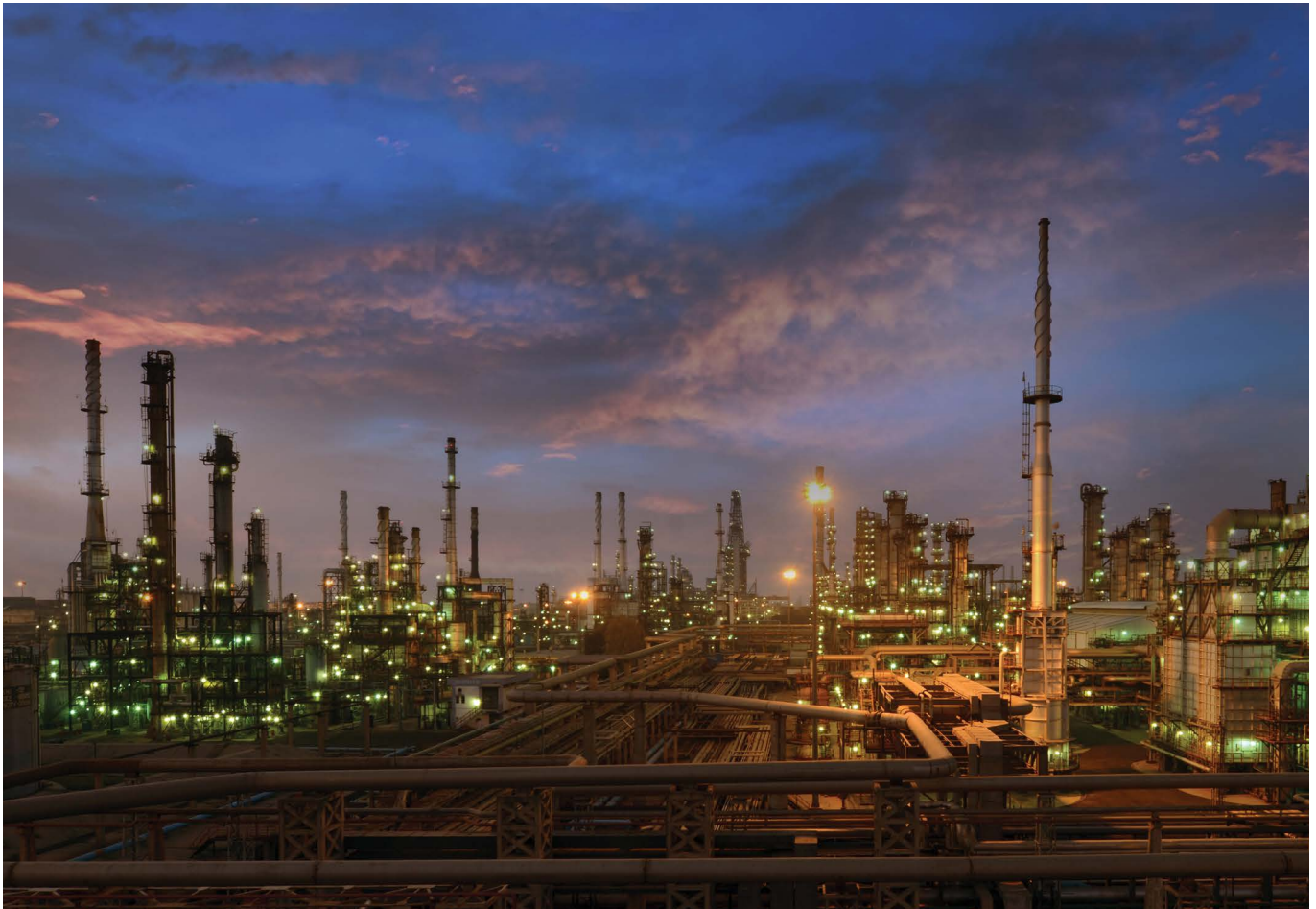
IndianOil refineries achieved a throughput of 69.42 MMT during FY 2019-20.
