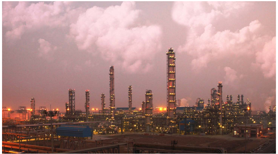
A view of IndianOil's Panipat Naphtha Cracker.
