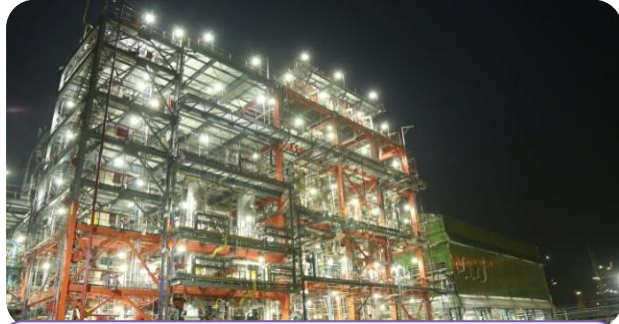
35 TMTPA INDAdapt G Plant at Guwahati Refinery
