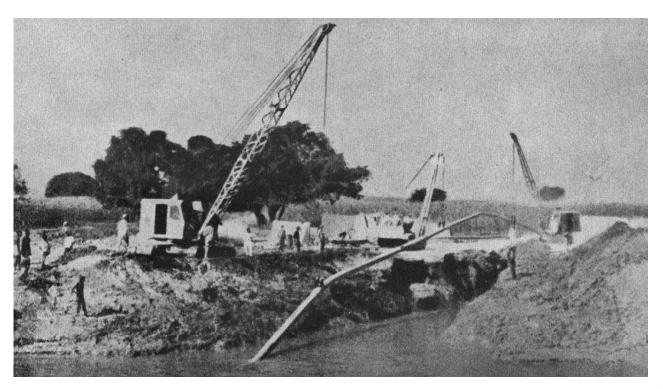
Pipelines traverse through hilly terrains and marshy areas. Picture shows work in progress at a submerged crossing.
