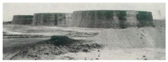
Pre-loading by sand of storage tanks at Haldia Refinery
