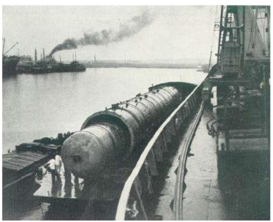
Crude distillation column for Haldia Refinery being off-loaded at Calcutta Prot
