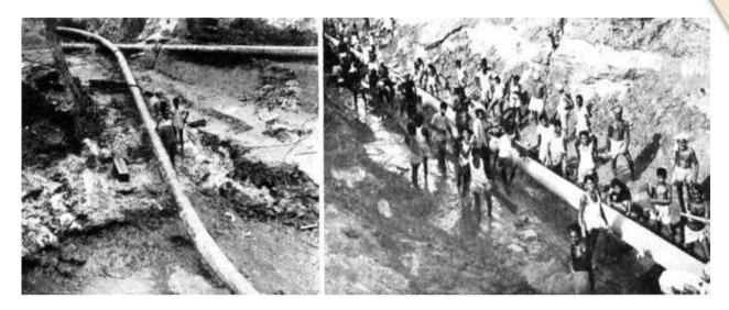
Diversion of Damodar River submerged crossing on Haldia-Mourigram Pipeline – lowering and diverting the pipeline.
