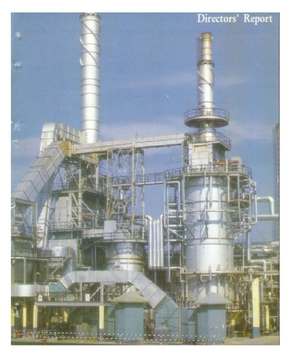
Atmospheric vacuum unit of Barauni refinery where secondary processing facilities have also been installed to meet the increasing demand of diesel, kerosene and cooking gas.
