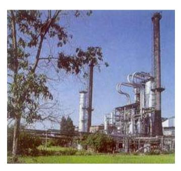
Digboi refinery commissioned a catalytic reforming unit during 1997-98 for production of low-lead and unleaded petrol
