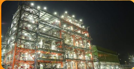
35 TMTA INDAdapt G Plant at Guwahati Refinery
