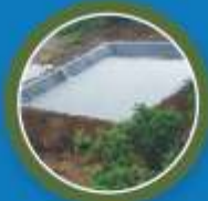
Rain Water Harvesting
