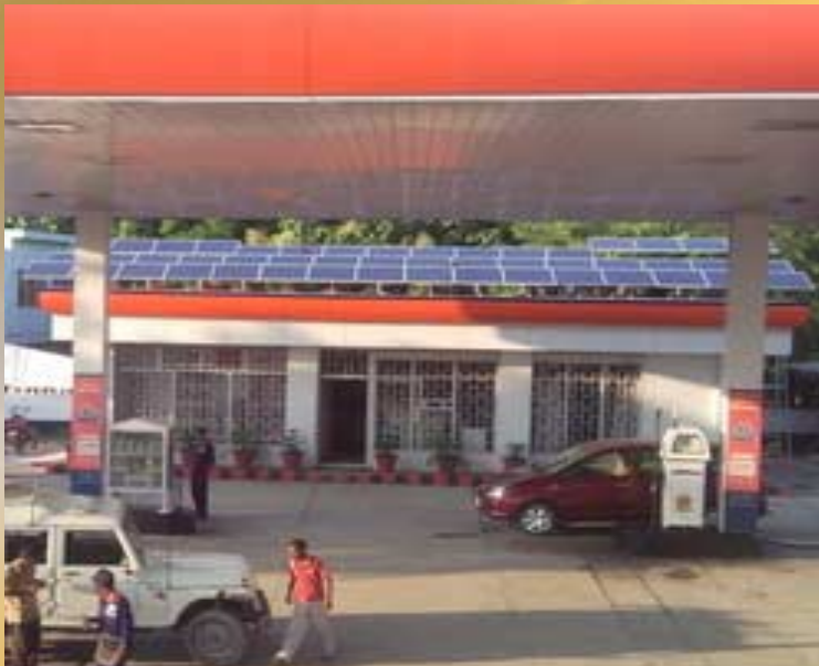
IndianOil RO with Rooftop Solar Panels
