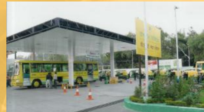
CNG Pump at Lucknow
