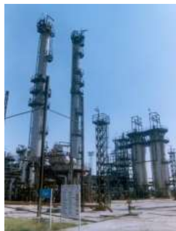
FGH Unit at IndianOil's Gujarat Refinery
