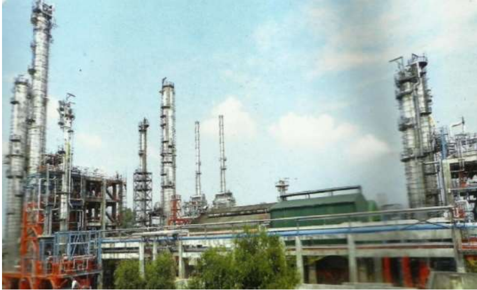
Naphtha Isomerization unit at Bongaigaon Refinery
