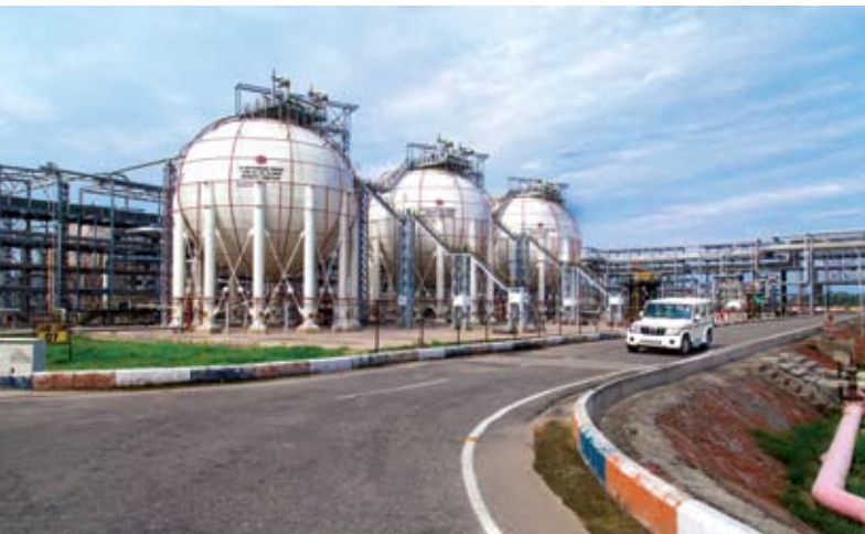
LPG Horton spheres at an Indane bottling facility.
