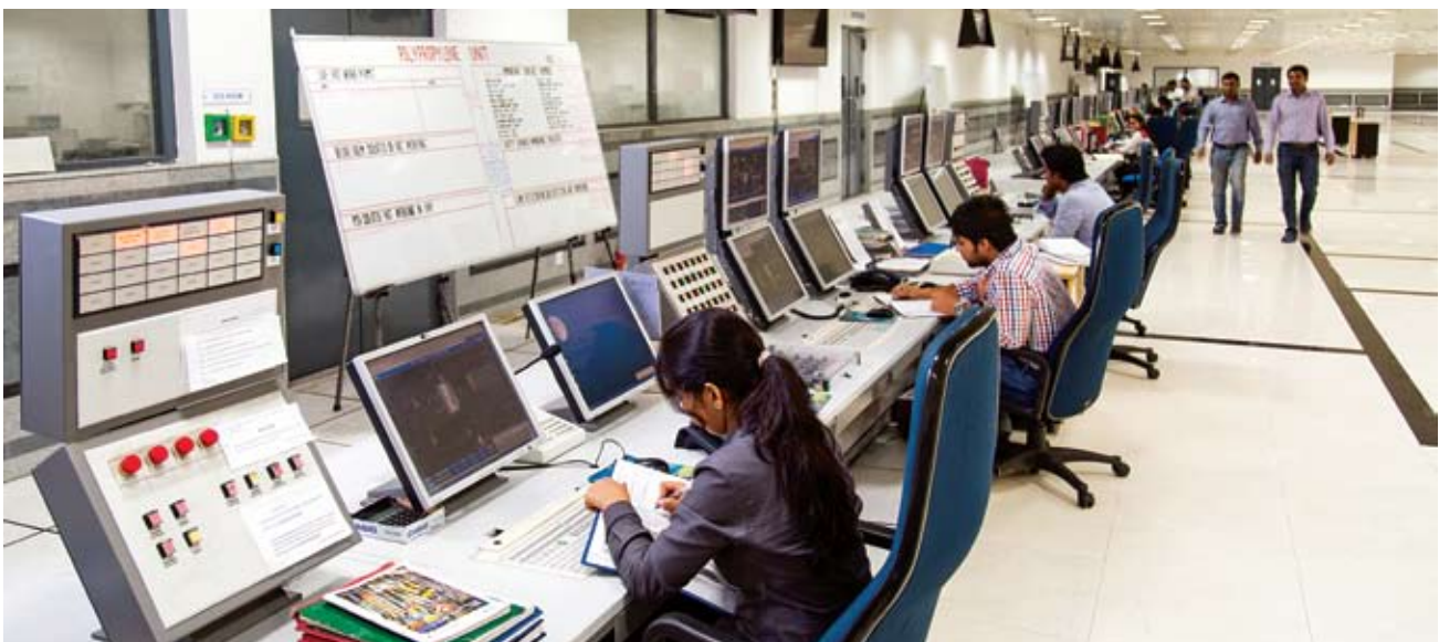
Young engineers manning the control room of the Paraxylene plant at IndianOil's Panipat Complex.
