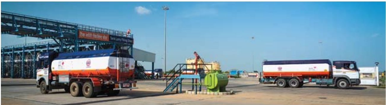
IndianOil's major grassroots petroleum bulk storage terminal commissioned at Mohanpura near Jaipur recently. The 'smart terminal' is fully automated with ultra-modern facilities.
