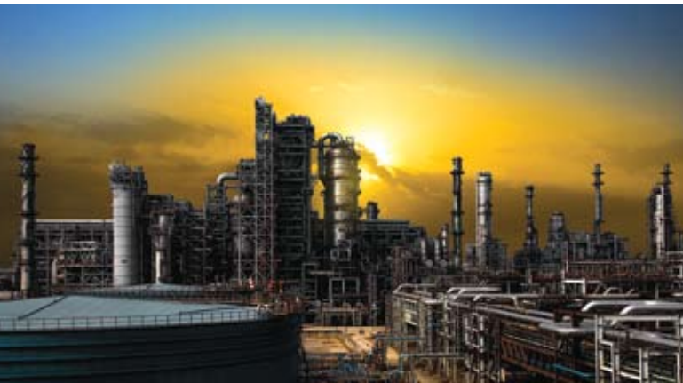
IndianOil's youngest refinery at Paradip: The Energy Gateway to East India.
