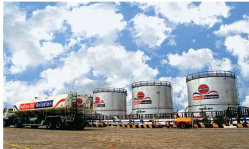
ATF storage tanks at an IndianOil aviation fuel station.
