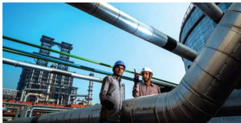
Pipelines at Paradip Refinery – lifelines to reach finished products to consumption centres.
