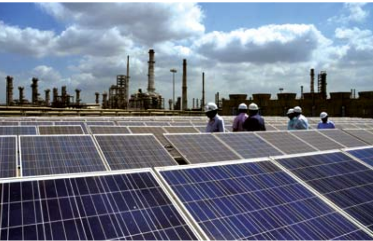
Solar energy farm at IndianOil's Koyali Refinery in Gujarat.
