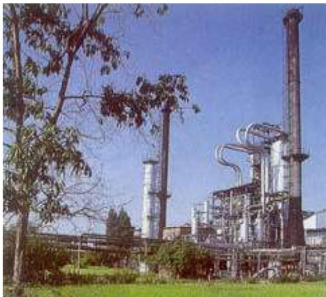
*Digboi refinery commissioned a catalytic reforming unit during 1997-98 for production of low-lead and unleaded petrol*
